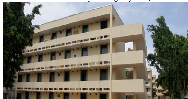
Figure 1.2: A picture showing the approach view of a block in the dormitory source; [24]
